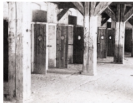
■ In the large spaces where rice was once stored before transport to Austria-Hungary, the narrow cells were created, the antechamber of the crematorium.
